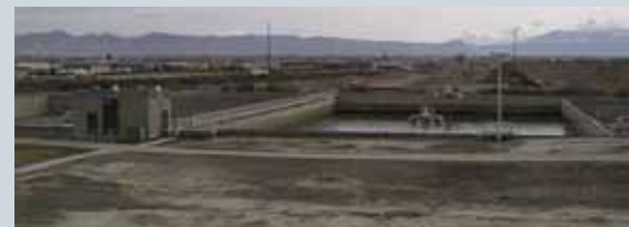
Persigo Waste Water Treatment Plant is a geographically large facility serving an even larger desert community.
